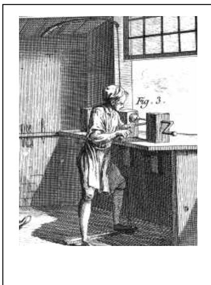
Fig.6. Button Maker using a spring pole lathe for buffing, or polishing buttons molded of resin.
