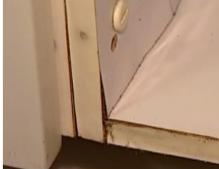
Figure 1 Wear of a piece of kitchen furniture of traditional construction
