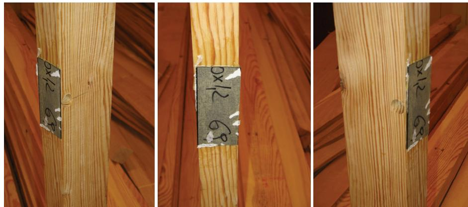
Fig. 1. Wooden beam reinforced locally with CFRP tape [5]
